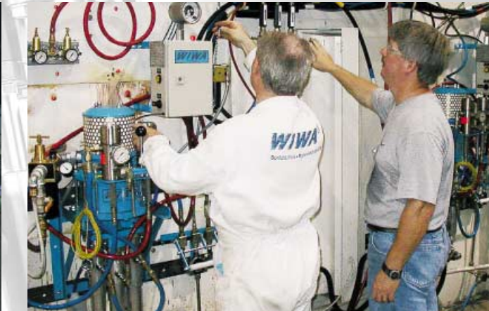
Commissioning a WIWA DUOMIX system in the United States
